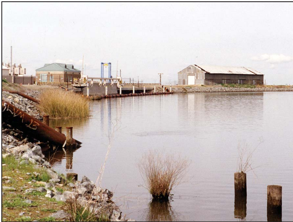
Photographs taken at the Old River Facility Pumping Plant, Los Vaqueros, California (Figure is for illustration purposes only.)
