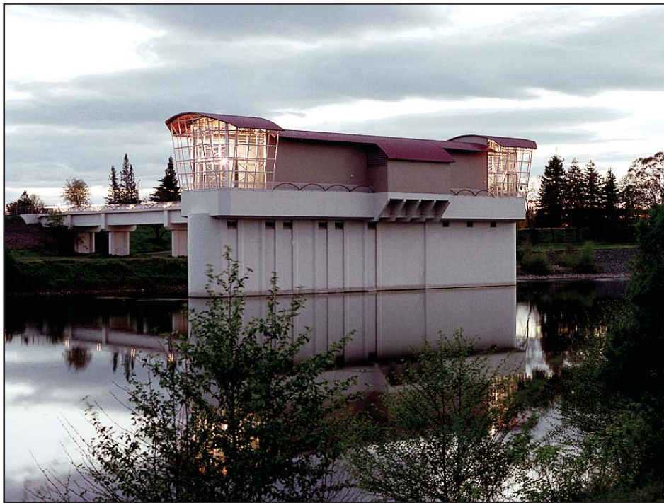
Photographs taken at the E.A. Fairbairn Water Treatment Plant in Sacramento, California (Figure is for illustration purposes only. Intake is 121 feet long, 30 feet wide, and 80 feet tall.)
